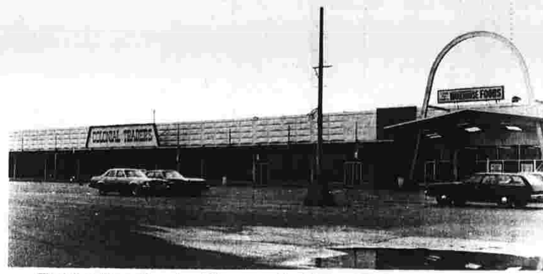
The former Topps Department Store, now site of Colonial Traders and part of Warehouse Foods, is the proposed location of a movie theater-restaurant. It will occupy a small portion of the large store off Main St. in East Hartford. (Herald photo by Barlow)
